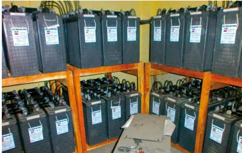
Fig.2. Battery Bank Installed to Store Solar Power
