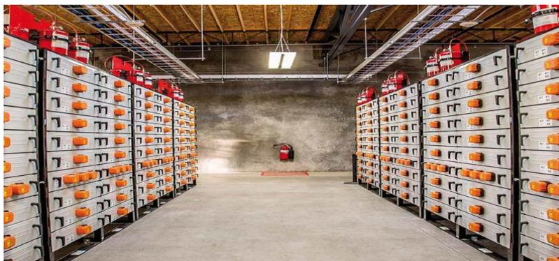
**Fig.1. A 5 MW Lithium-Ion Energy Storage System**
